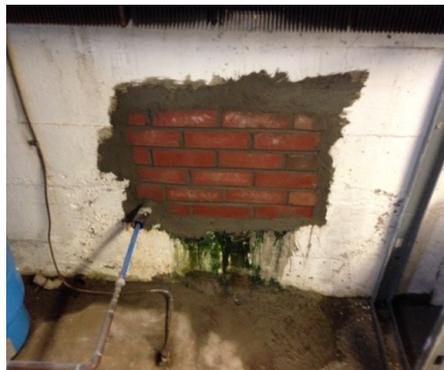
After: Foundation hole bricked in by contractor Jason Knight.
