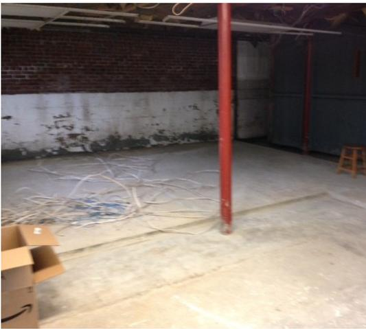
View showing higher cement floor to be removed before new floor is poured.
