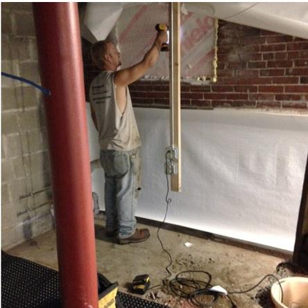
Drain line opening for commercial dehumidifier being drilled by T.C. Hafford's Colby.
