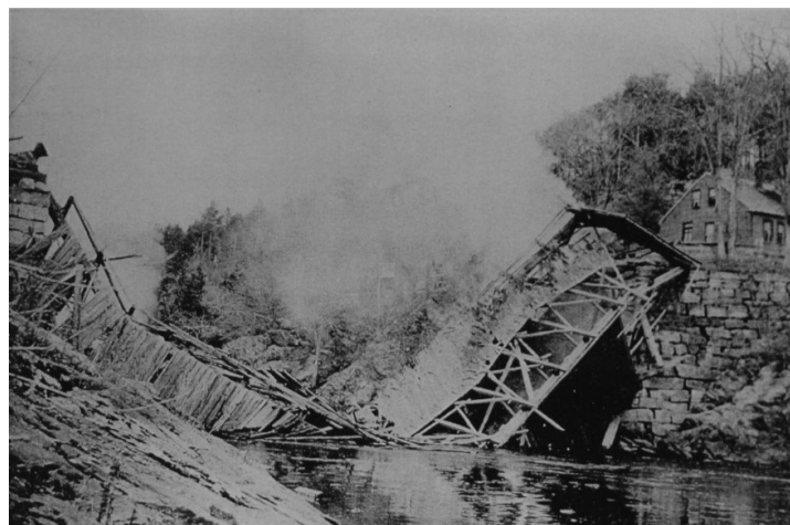
Demolition of the old Union Falls Bridge
